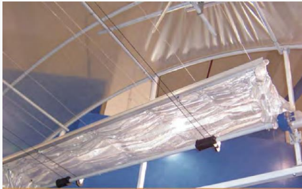
a. Application on Screening System
